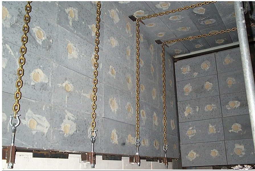
Refractory lined burn chamber
